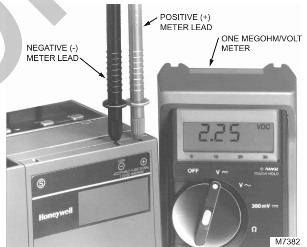
Fig. 17. Flame signal measurement.
